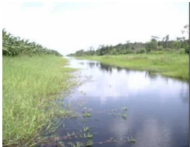
The Stondansie irrigation canal, relatively clean but locally overgrown.
