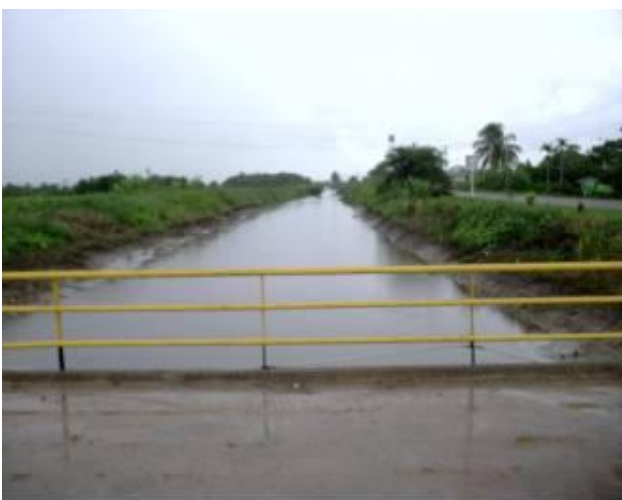
A clean drainage canal at the Henar polder.
