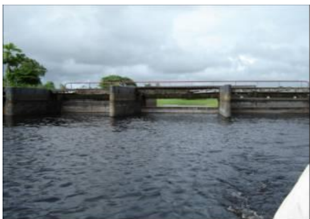
Weir at the Nanni inlet. This weir allows excess water to flow through the Nanni creek to the Corantijn river. Operation of this weir is always a problem.
